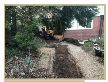
drainage works underway. Currently none of the groundwater (on the steep slope on which the presbytery is located) or roof run-off water is captured leading to on-going mildew problems in the house, inability of present guttering to cope with overflow and all water draining ultimately onto the neighbour's property. current works will capture all roof run-off and groundwater flow and drain it to the street.
